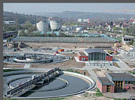
Main Sewage Treatment Plant Stuttgart 1.2 Mio PE, Germany
