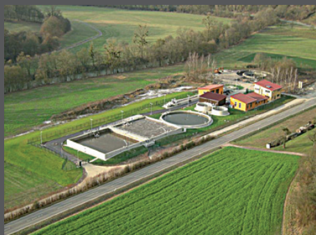
Sewage Treatment Plant Widdern 16.000 PE, Germany
