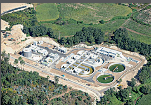
Sewage Treatment Plant Sousa 90.000 PE, Portugal
